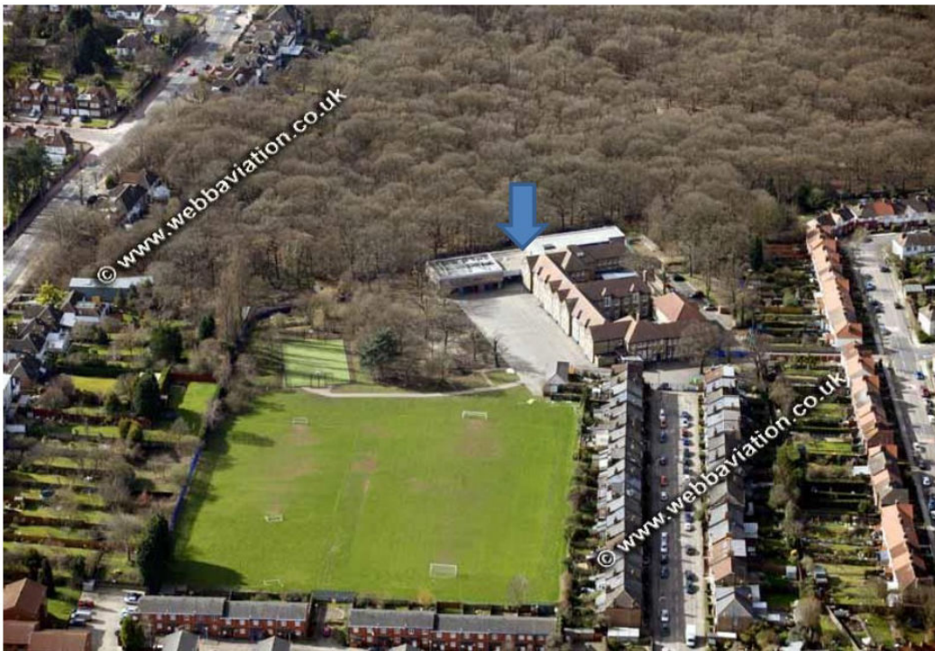
Aerial Photo of the site with location of new music room arrowed
