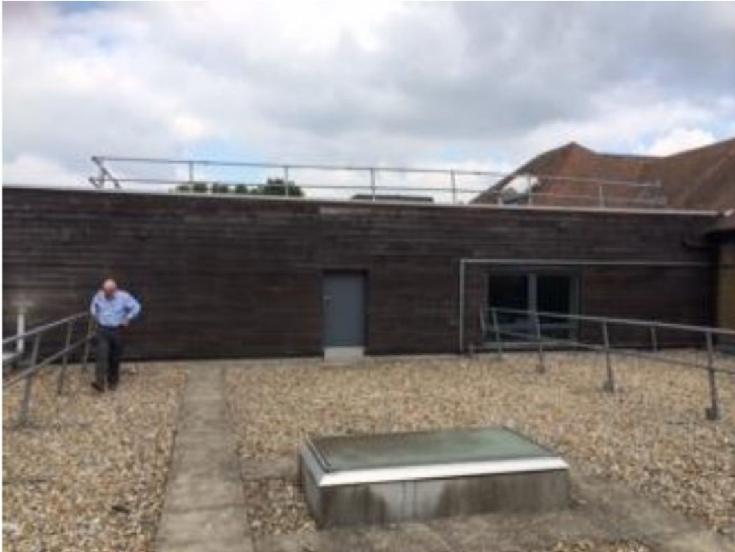
Roof deck location for extension looking north
